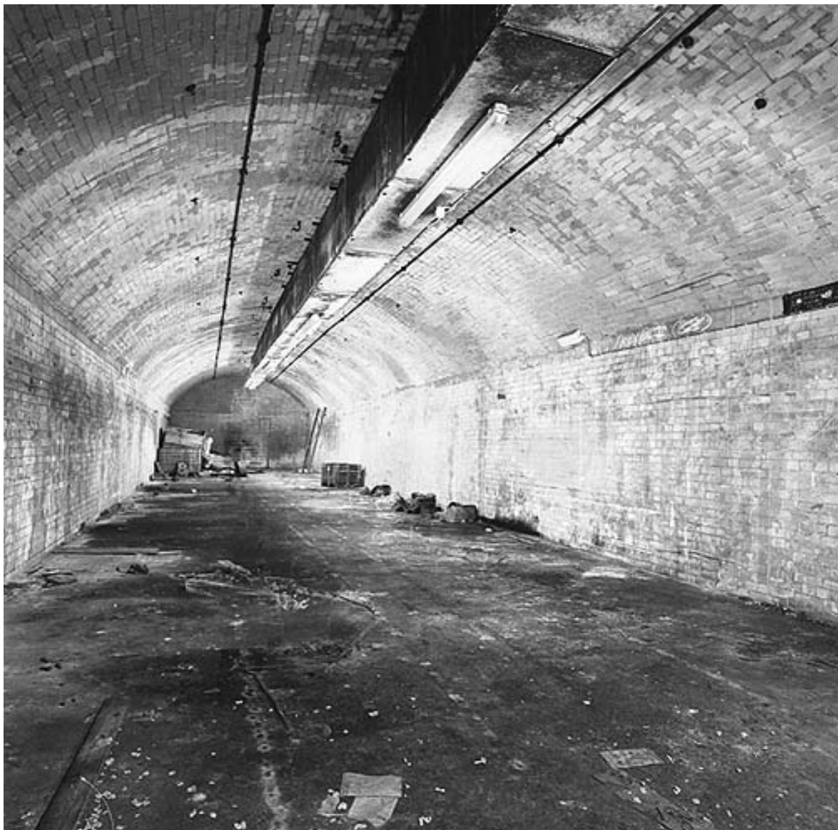
One of the 100 metre factory tunnels - Nick Catford
